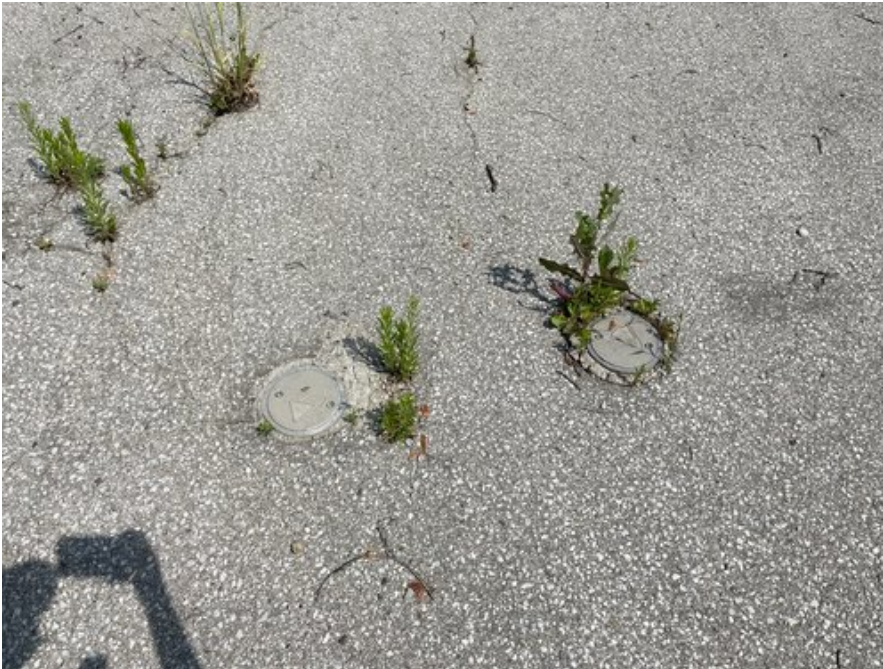
7. Monitoring wells from previous 2018 Phase One ESA.
