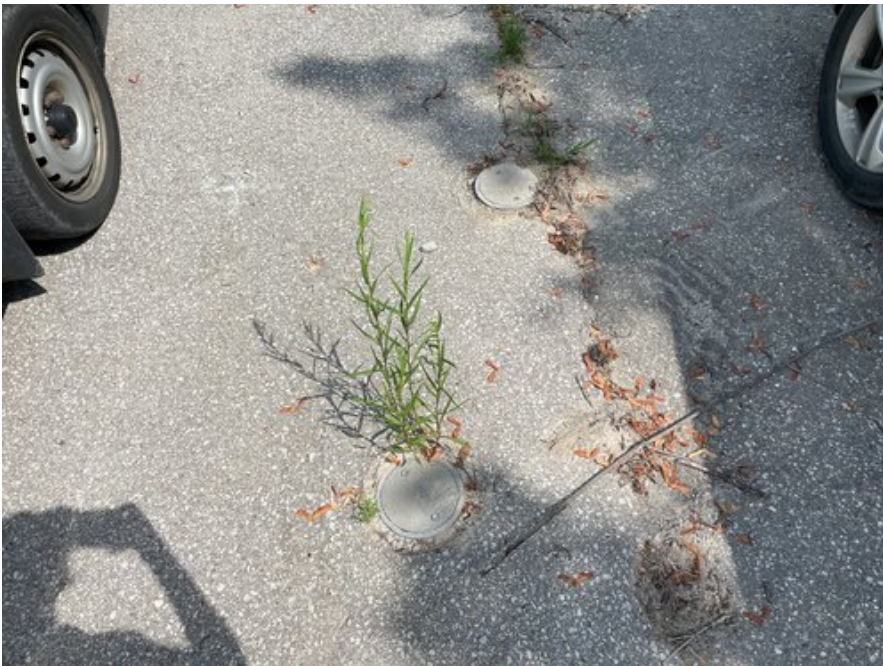
4. Monitoring wells from previous 2018 Phase One ESA.
